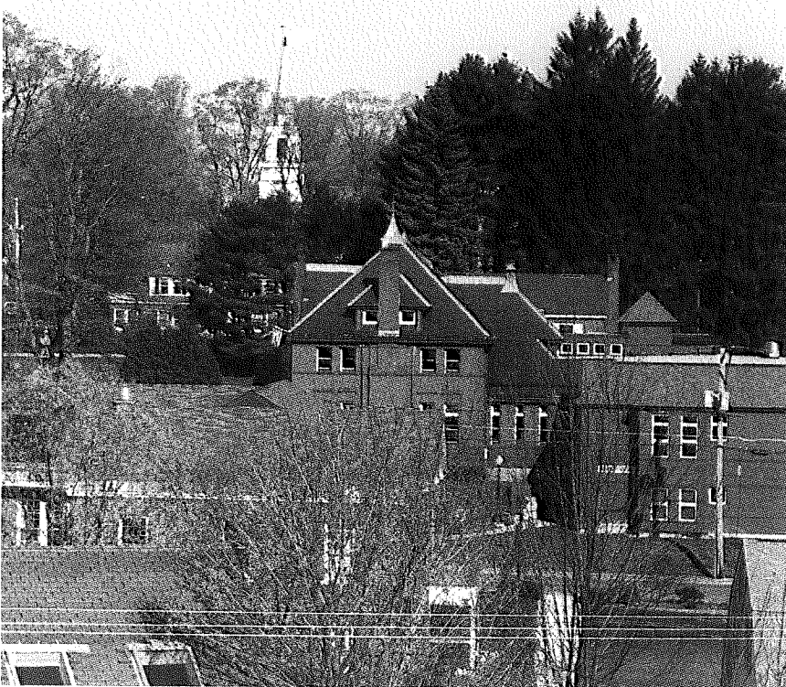
1-24 Looking west from atop the Granite State Hotel. Beyond the Monadnock Bank is Dr. O. H. Bradley's house (see Nos. 1-25 & 1-26) and the East Congregational Church (United Church). In 1896 the Library was sited on land obtained from Bradley; and seventy years later, in 1966, the house itself gave way to the Civic Center. The bank building shown here, the third one after two disastrous fires, was built in 1878. The modern view was taken from the roof of the Jaffrey Mills. Note the stone wall along what is now Goodnow Street; it may have been removed when the library was built. Between 1879 and 1882.
