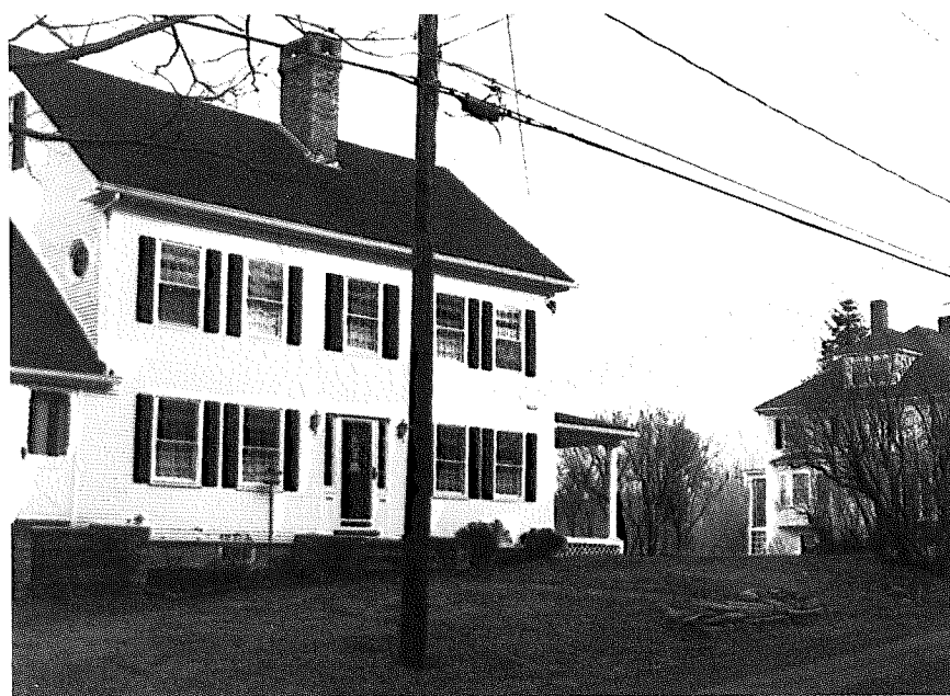
4-12 "The Farmhouse," South Hill Road. For his labors as minister, Laban Ainsworth received in addition to a housesite land for farming purposes. He built this farmhouse across from The Manse in the early 1800s and rented it out to supplement his income. Originally the house was one and a half stories; it was later raised with a new story built underneath. The earlier view shows a classic connected New England farm complex: "big house, little house, back house, barn." The barn was relocated further down South Hill Road when the "Colonial" was built in 1910-11. The Farmhouse has within recent years been extensively renovated. Prior to 1910.
