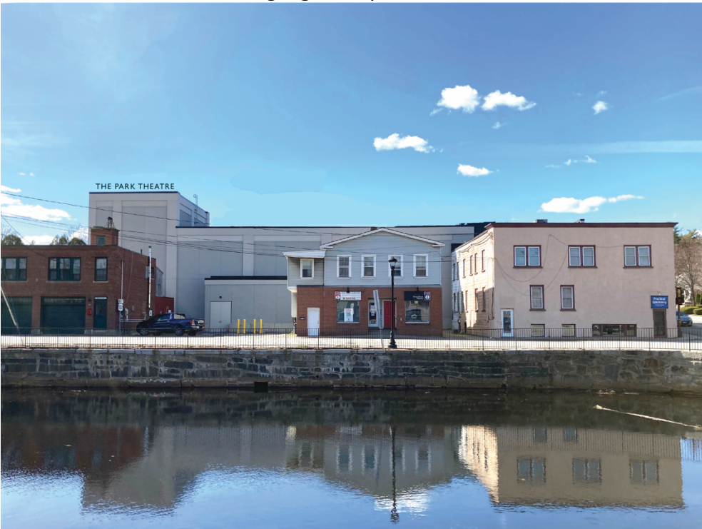
Signage on flyloft roof
