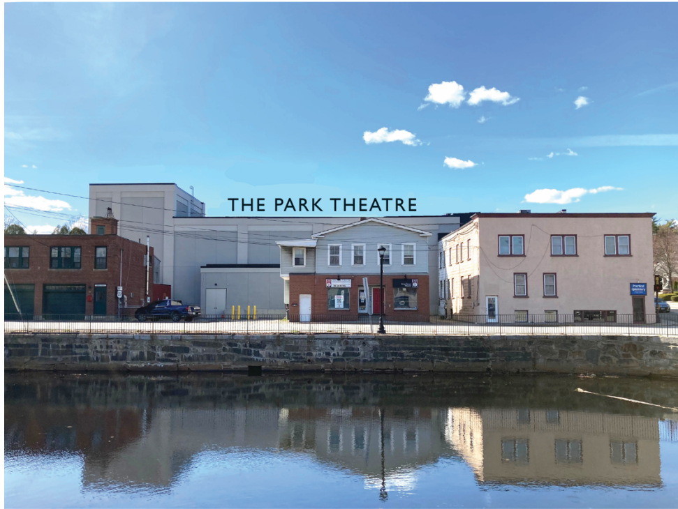
Signage on auditorium roof
