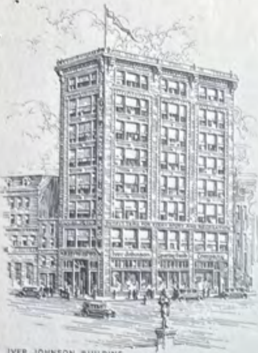
IVER JOHNSON BUILDING
