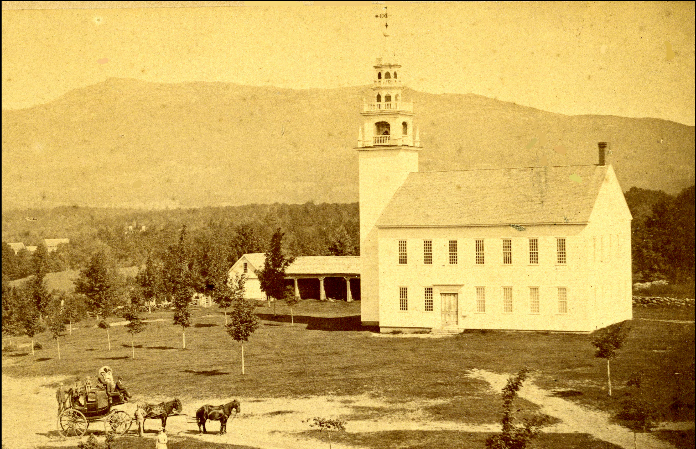
The Meetinghouse. Location of Town Meetings from 1775-1914. Town offices on second floor from 1870 to 1896.
