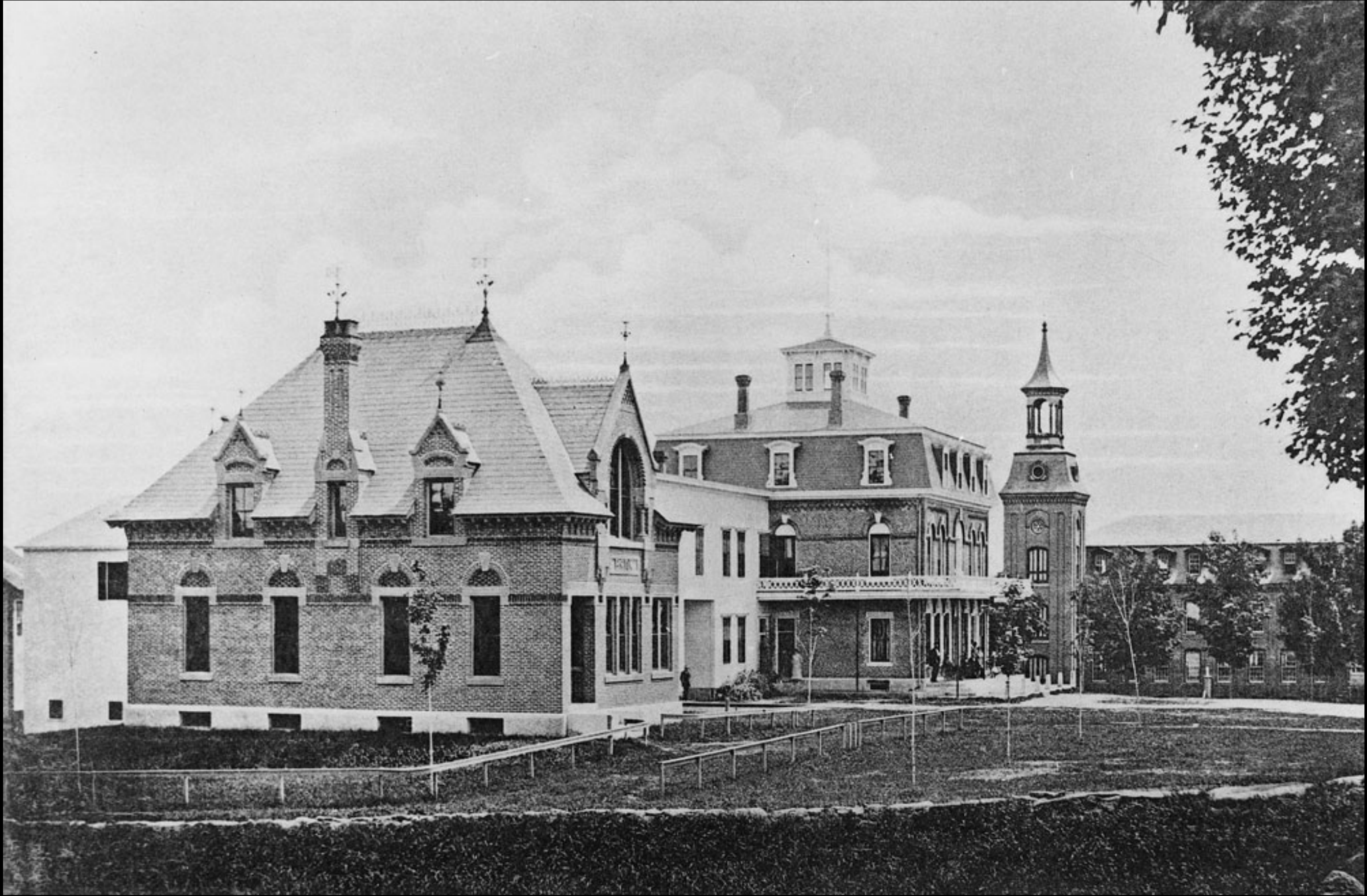
Monadnock Bank, Granite State Hotel and the Jaffrey Mills. Ca. 1880.
