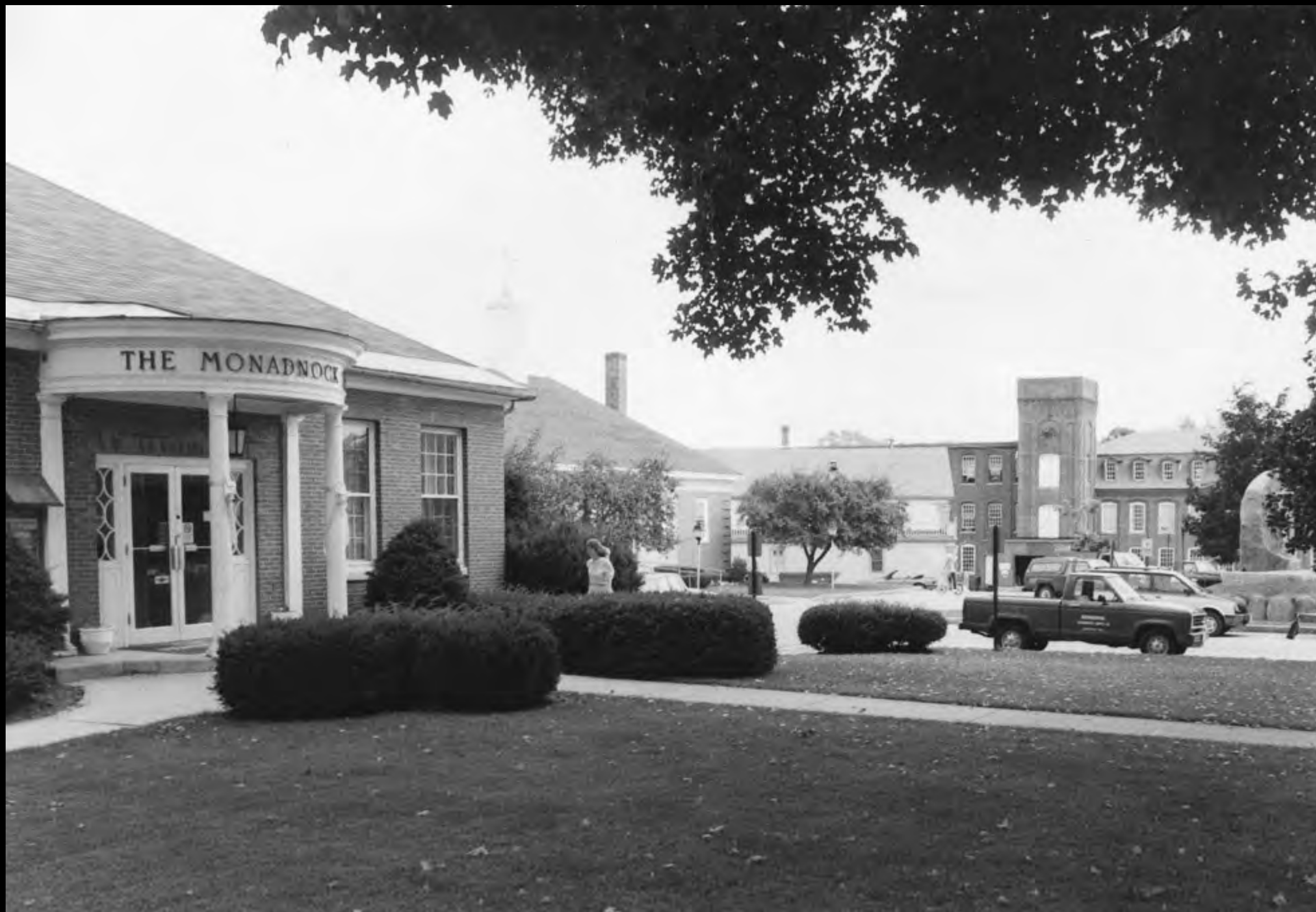
Monadnock Bank, Town Offices and the Jaffrey Mills, 1994.
